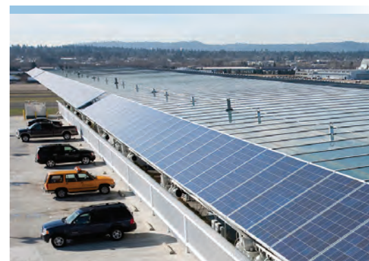
Nike, Delta Air Lines, and the Port joined forces to install solar panels on the Airport's canopy
